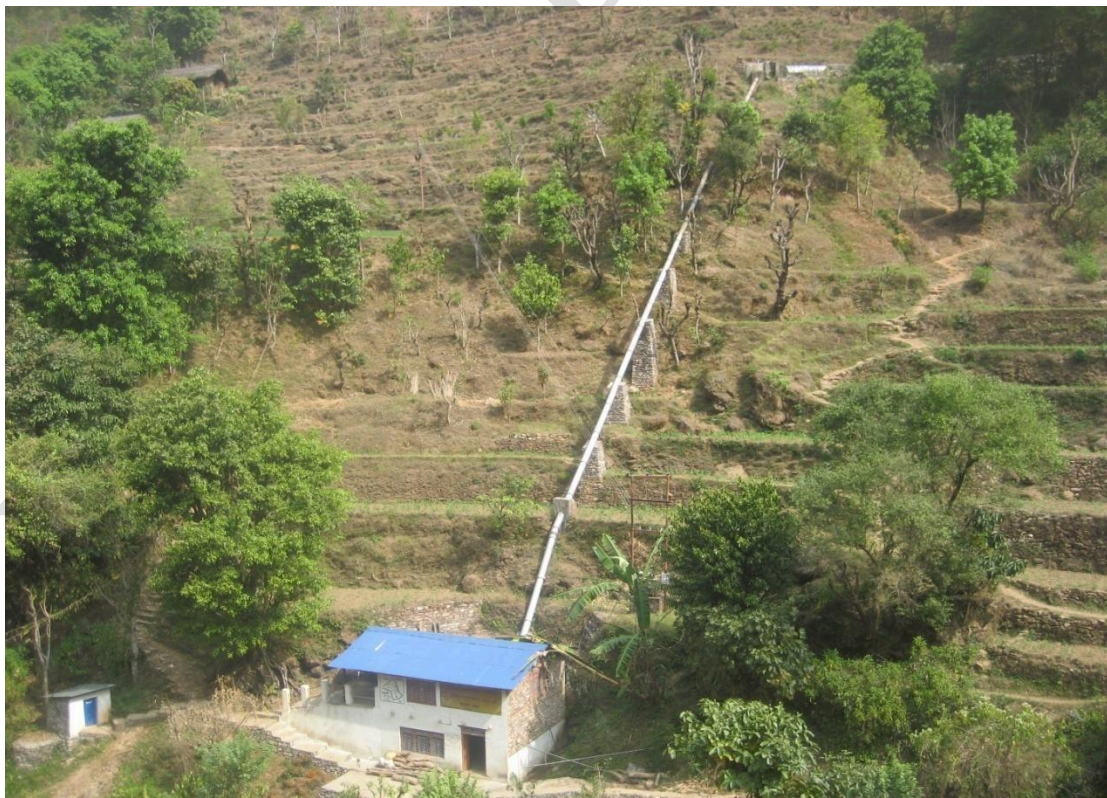
Penstock Alignment and Power house
