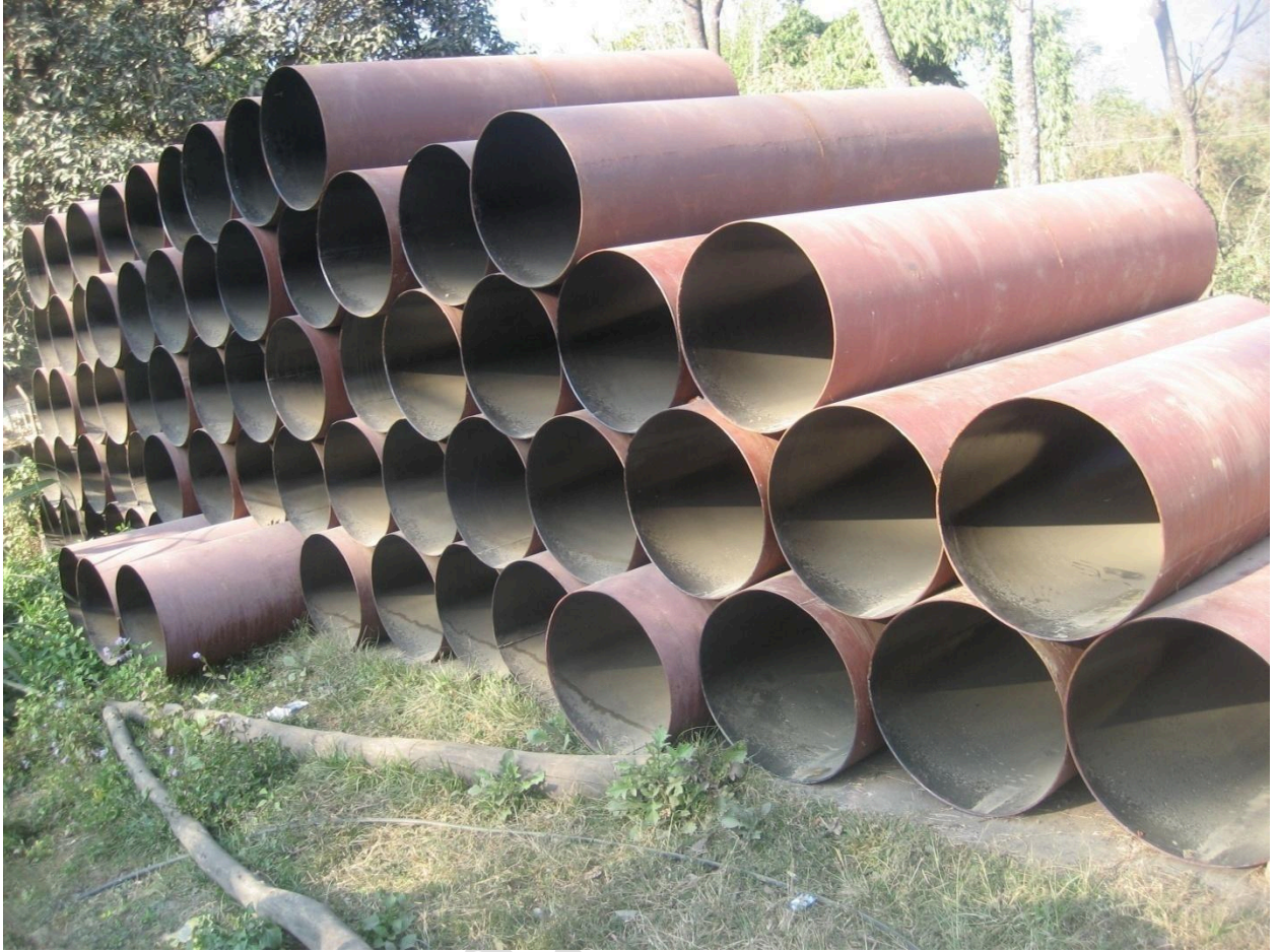
Penstock pipes ready for transport
