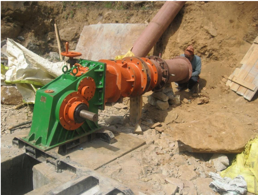
Installation of Cross flow Turbine at site – 92 KW, Achham
