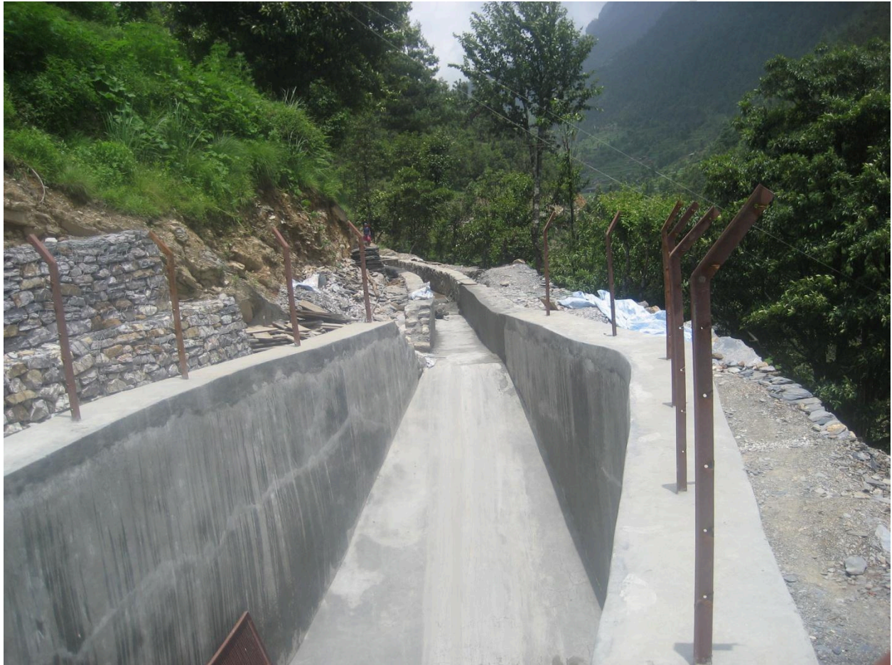
Forebay Tank of Tara Khola community Mini HEP (500 KW), Tara, Baglung
